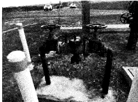
RPBP 25, Intersection of Kala Rd & Haleakala Hwy inside bollard perimeter
