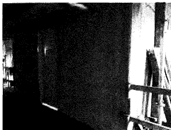
RPBP 48, outside Trash Room along wall near elevated platform
