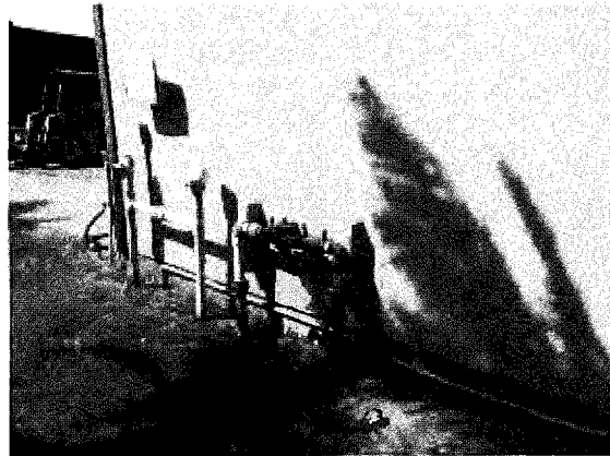
RPBP 18, Outside east-most building of Nursery, inside fenced area against building
