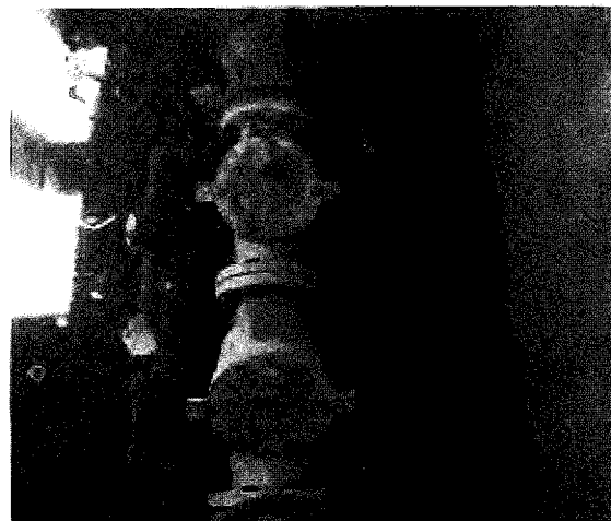
RPBP 19 & 20, Outside Maintenance Baseyard in concrete vault
