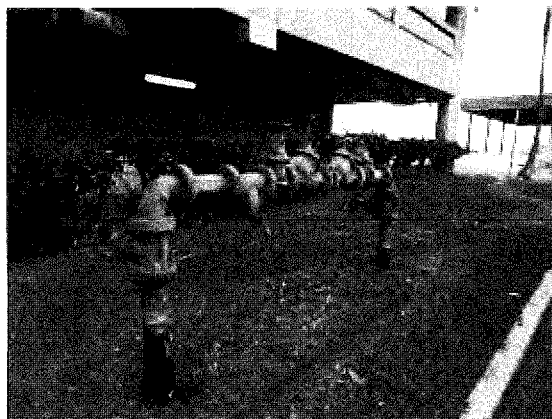
RPBP 46, outside chiller room in gravel area
