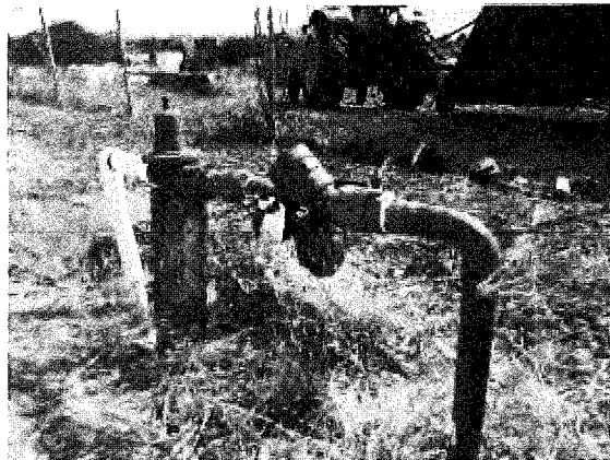
RPBP 17, Inside fenced area, south side of baseyard
